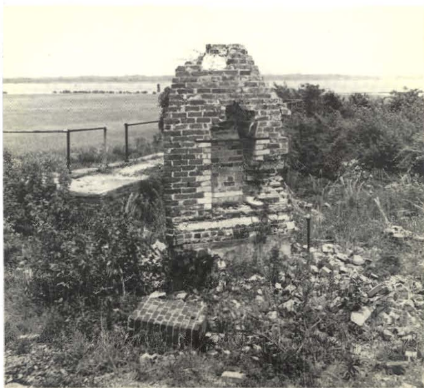
FIGURE 32. Chimney of light station building.
