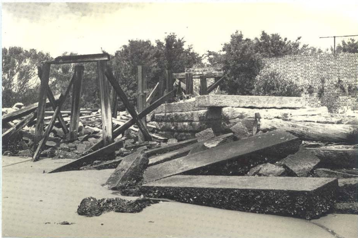
FIGURE 36. Photograph of remains of stone wharf.
