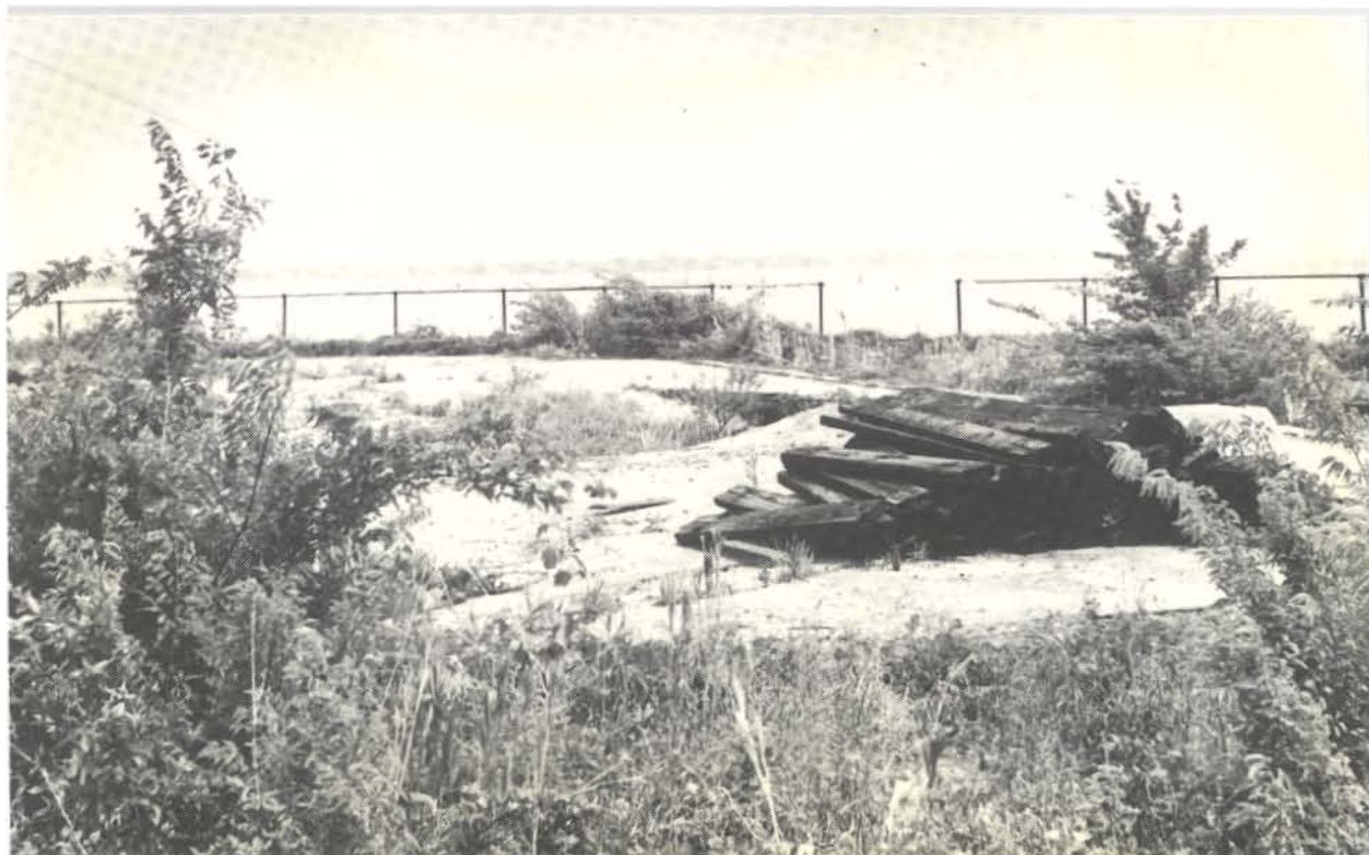
FIGURE 31. Photograph of light station ruins.
