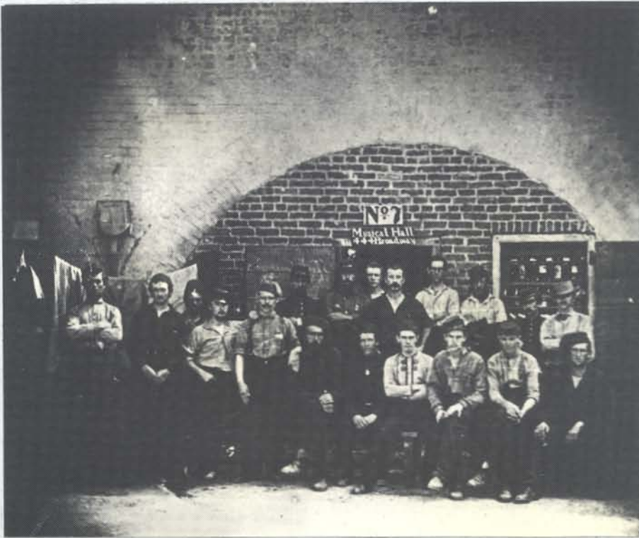
FIGURE 15. Photograph of prisoners from the United States 69th Regiment outside one of the bricked up casemates at Castle Pinckney (Courtesy Charleston Evening Post - The News and Courier ).
