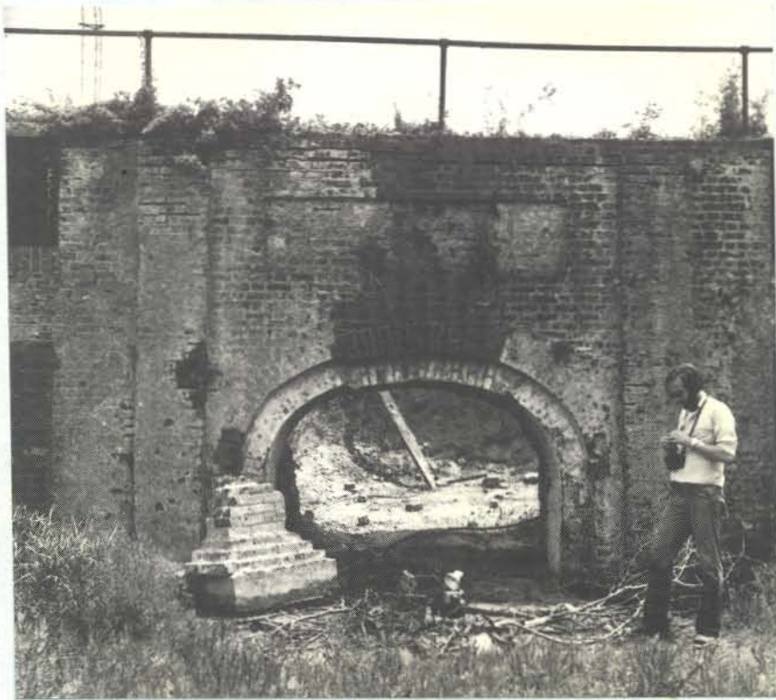
FIGURE 30. Photograph of Castle Pinckney gate from the outside showing ground level, vegetation and Castle Pinckney's subsidence.
