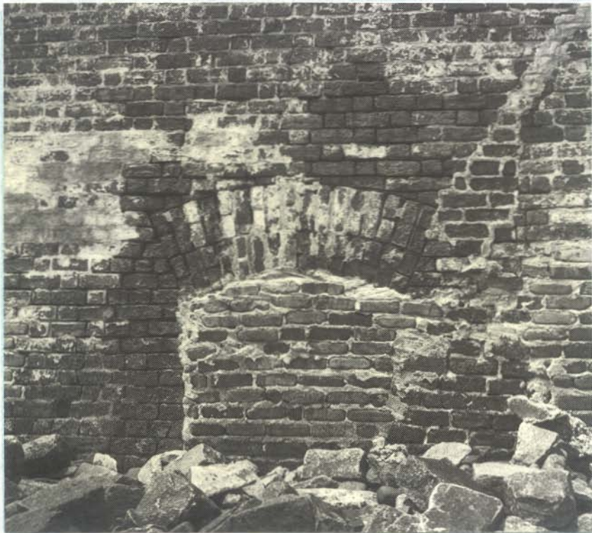
FIGURE 39. Wall of Castle Pinckney showing bricked up embrasures and efflorescence.
