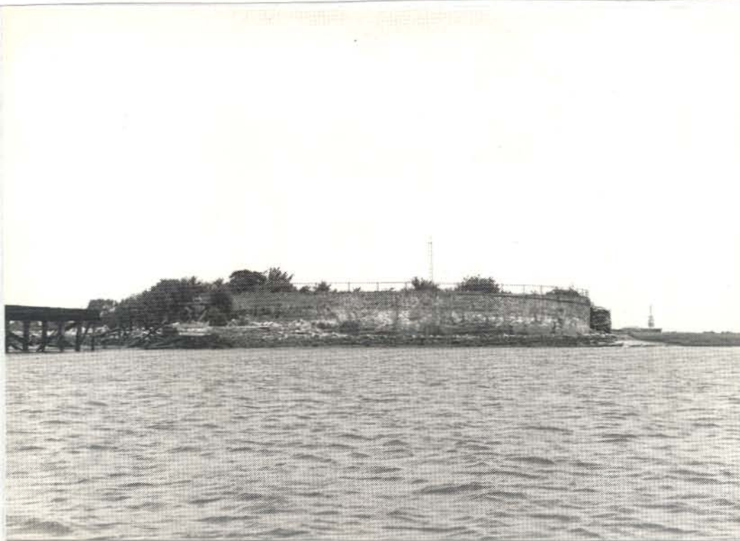
FIGURE 2. Southeastern approach to Castle Pinckney in the Cooper River.
