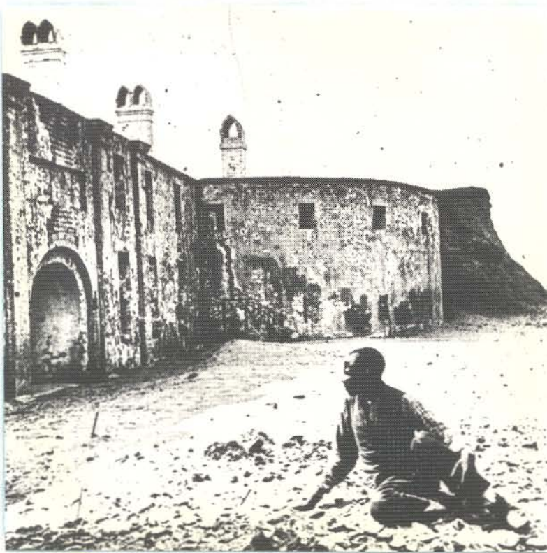
FIGURE 27. Post war photograph of gorge wall of Castle Pinckney showing the earthworks in cross section. The deteriorating condition of the brickwork can be seen. The embrasures had not been bricked up at this point. (Courtesy Charleston Evening Post - The News and Courier).
