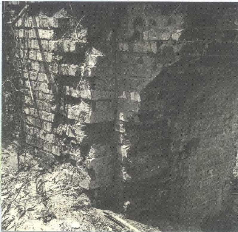
FIGURE 35. Close up photograph of rear barracks wall and a portion of the main gate.
