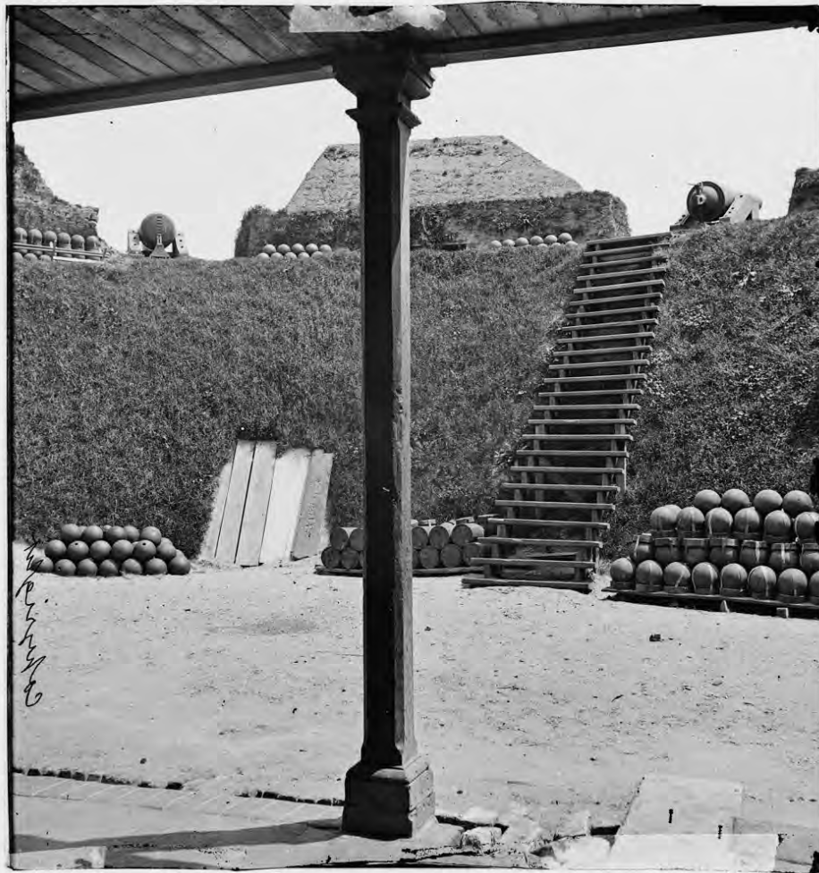
Figure 4: An Interior photo taken of Castle Pinckney in 1865 where earthworks, a 10-inch Columbiad, and a 7-inch Brooke Rifle can be seen in the background. (Photo courtesy of Library of Congress, www.loc.gov/item/2018666905/ )
